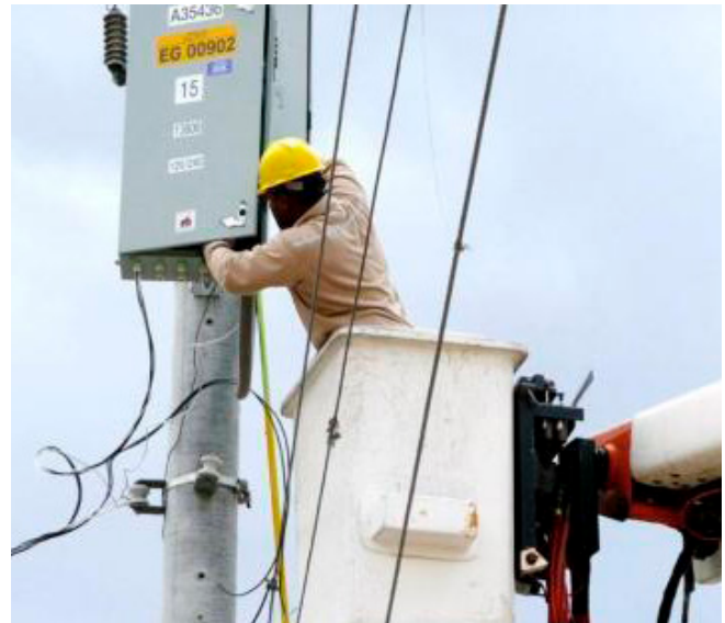
A JPS lineman on the job.
