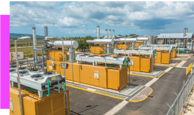
A view of the JPS 10MW Combined Heat & Power (CHP) Plant providing electricity and steam to the CB Group's processing plant.
