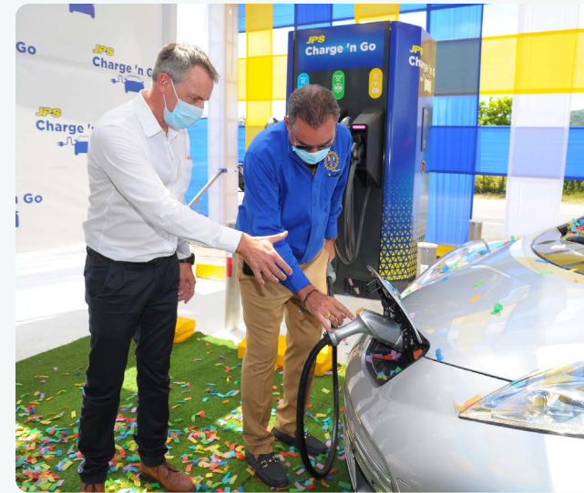
JPS COMMISSIONS ITS FIRST CHARGE N GO STATION: Minister of Science, Energy and Technology, Honourable Daryl Vaz (right) and JPS President & CEO, Michel Gantois, get the hang of using the electric vehicle charger at the Boot Gas Station in Drax Hall, St. Ann.
